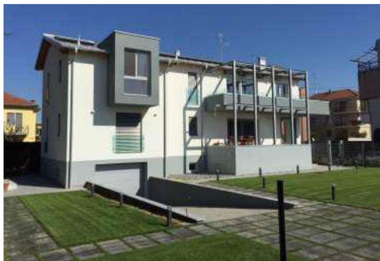
Figure 1. South-facing facade of the reference building.
