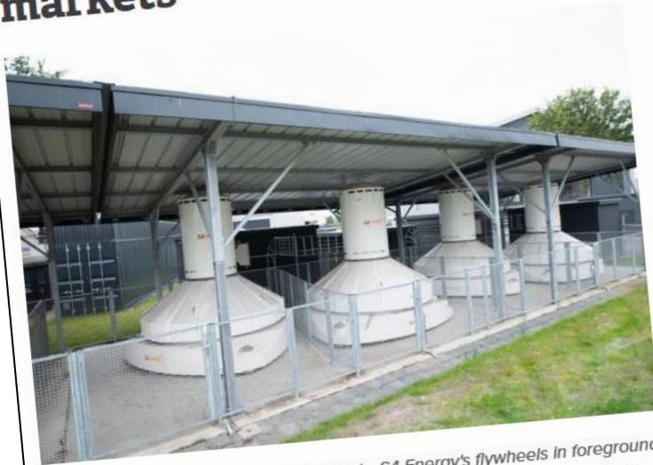
The hybrid system in Almelo, Netherlands. S4 Energy's flywheels in foreground with Leclanché containerised battery storage systems behind. Image: Leclanché.
